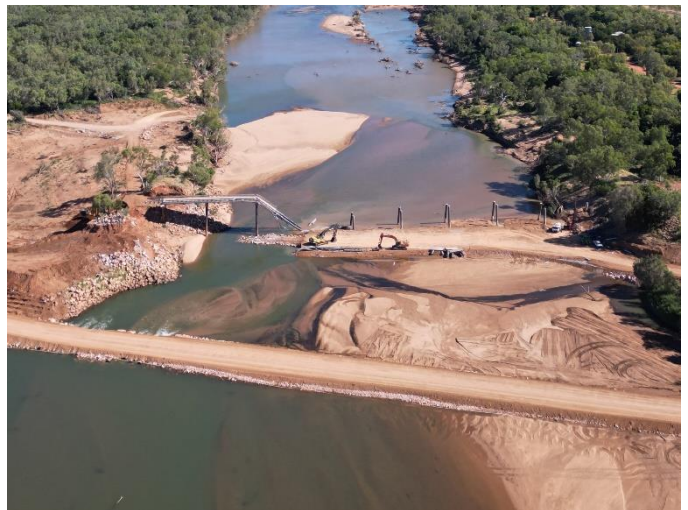
Demolition of the old Fitzroy River Bridge.
