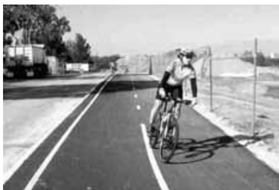
Temporary Path Surface A
