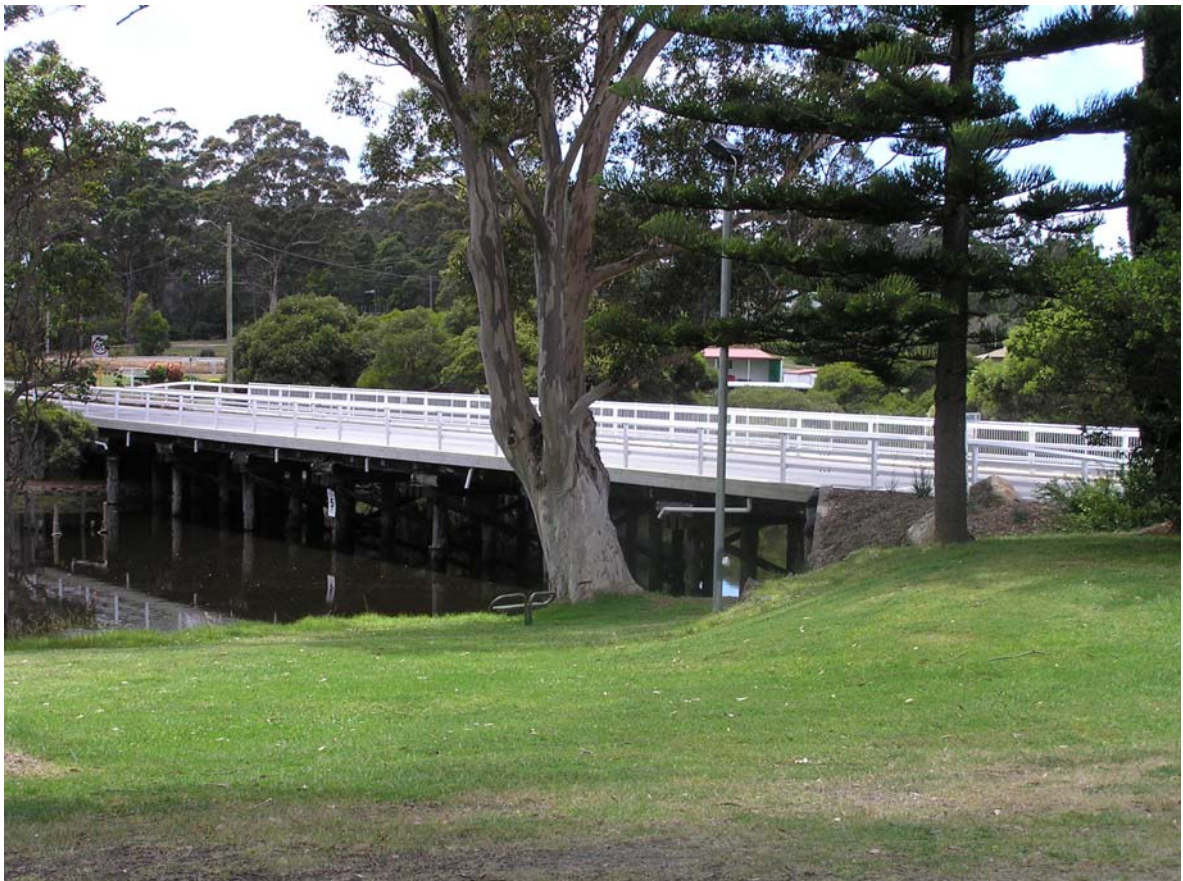
Denmark River Bridge No. 86A
