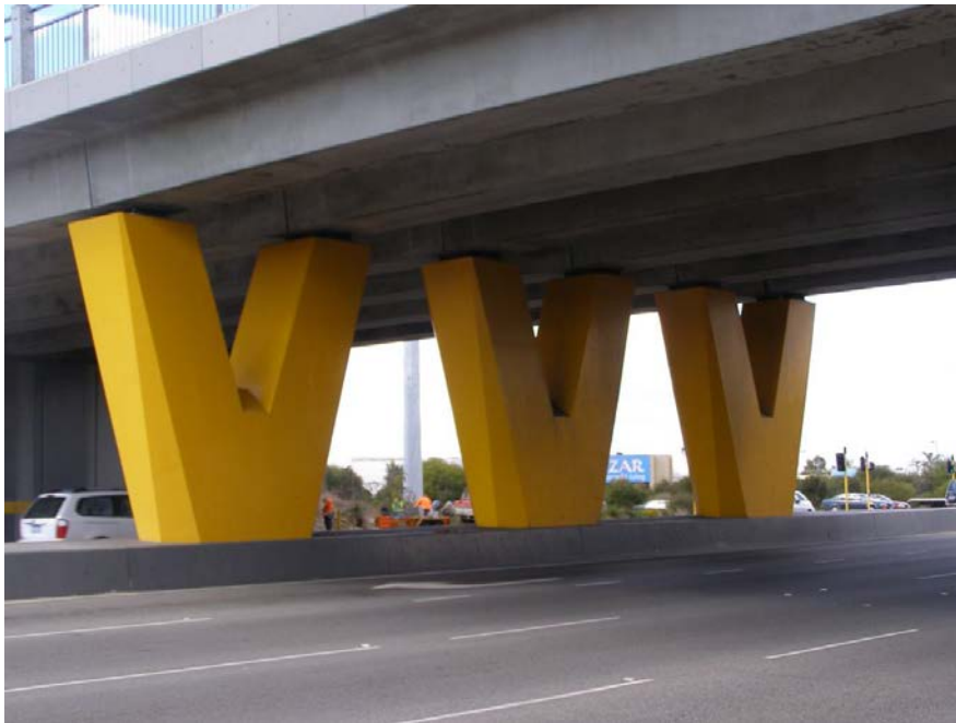
Figure 22.8 – TEEROFF BEAMS CONTINUING OVER THE PIER
