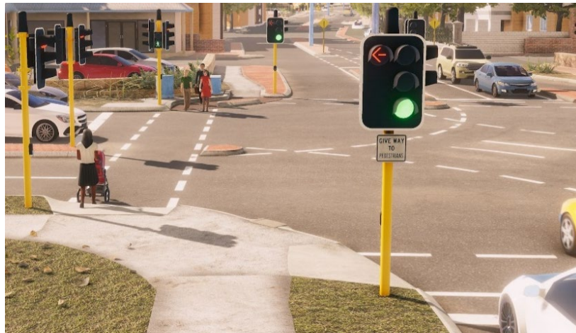
Image 7: Six seconds Invitation-to-Cross for pedestrians
