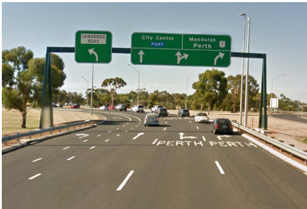
Figure C.3: Eelup Rotary showing Overhead Advance Direction Signs and Supplementary Pavement Markings
