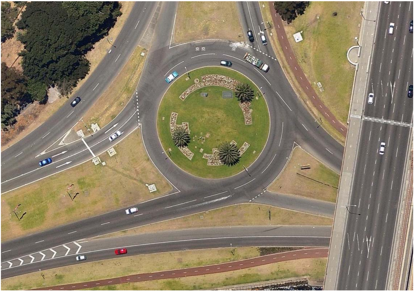
Figure D.2: Point Lewis Rotary after Installation of Roundabout Metering Signals
