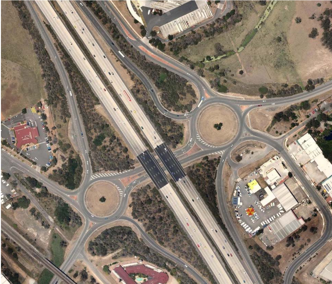
Figure A.3: Example of Two Multi-lane Roundabouts with more than Four Legs
