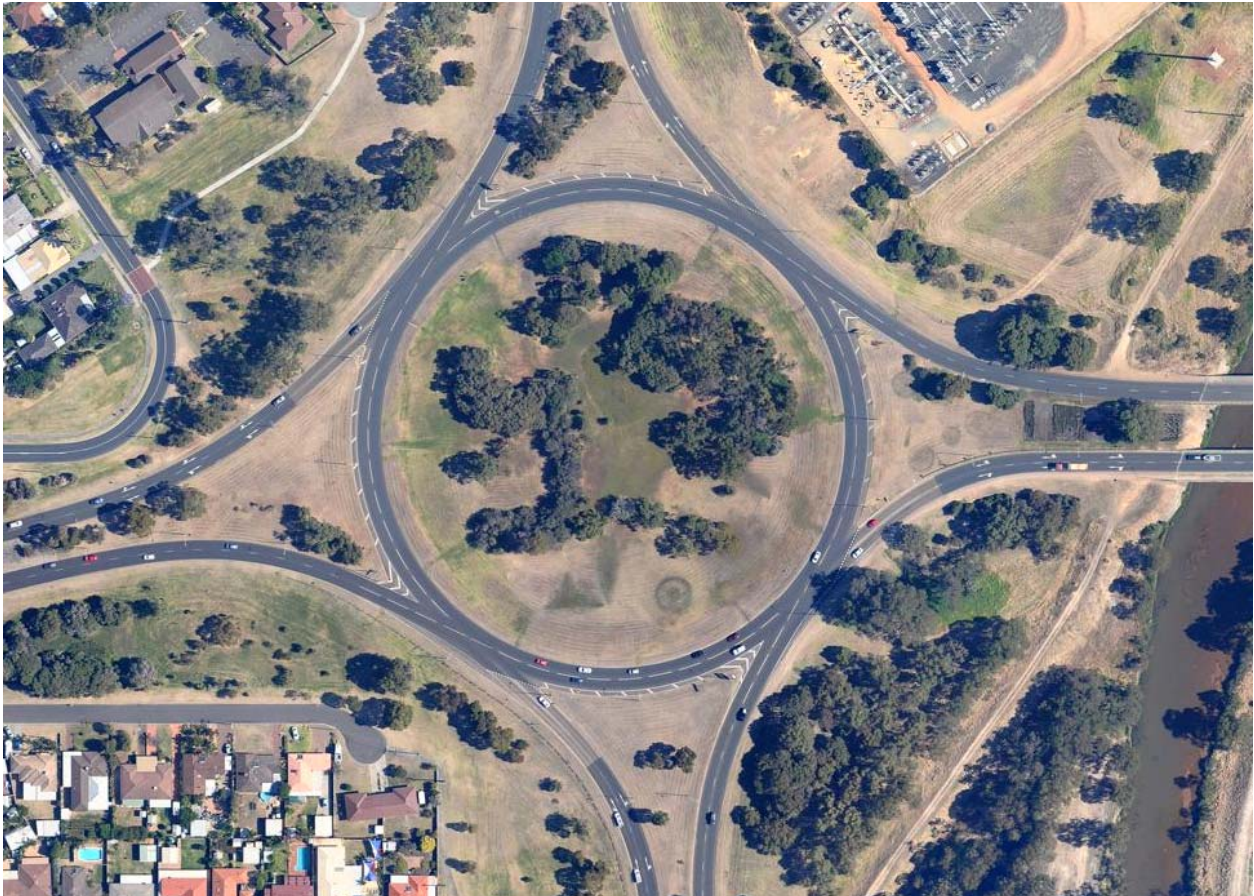
Figure C.1: Eelup Rotary in 2011 prior to Upgrading
