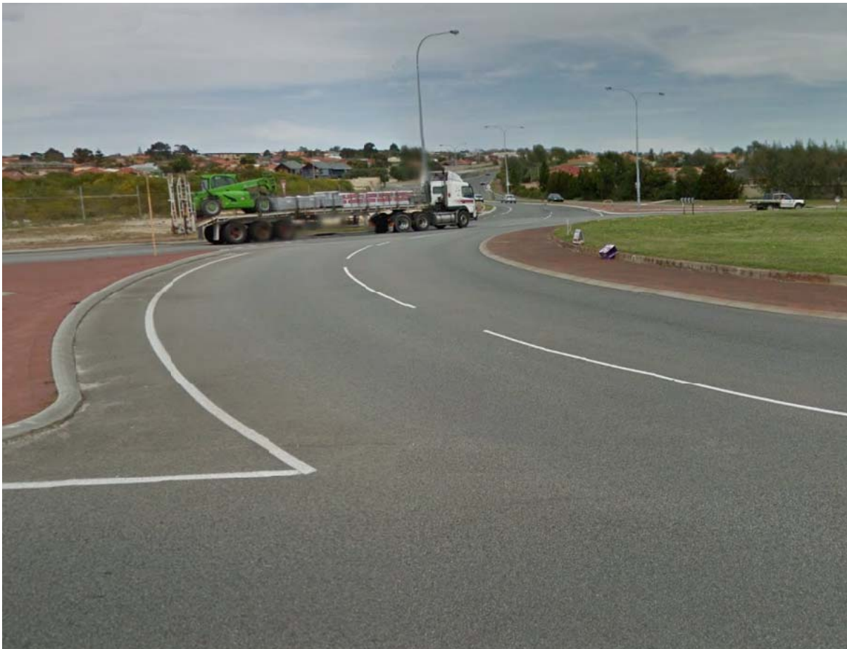
Figure 4.4: Example of a Heavy Vehicle Apron Around the Central Island of a Roundabout
