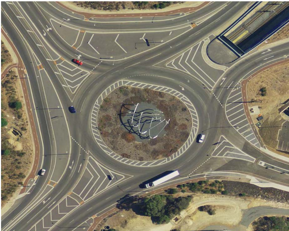
Figure C1.5 Example of “Spiral” Markings on a Roundabout in Mandurah to Facilitate Double Right Turns
