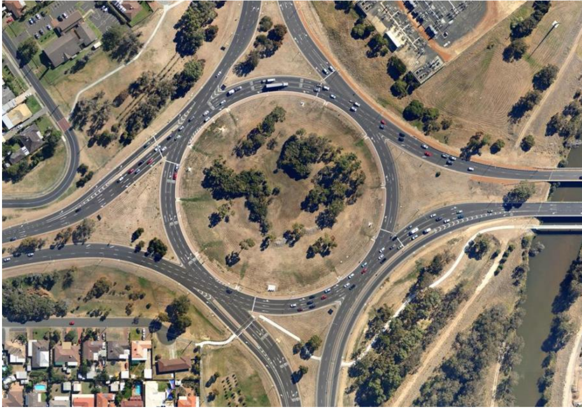
Figure C.2: Eelup Rotary in 2014 after Upgrading
