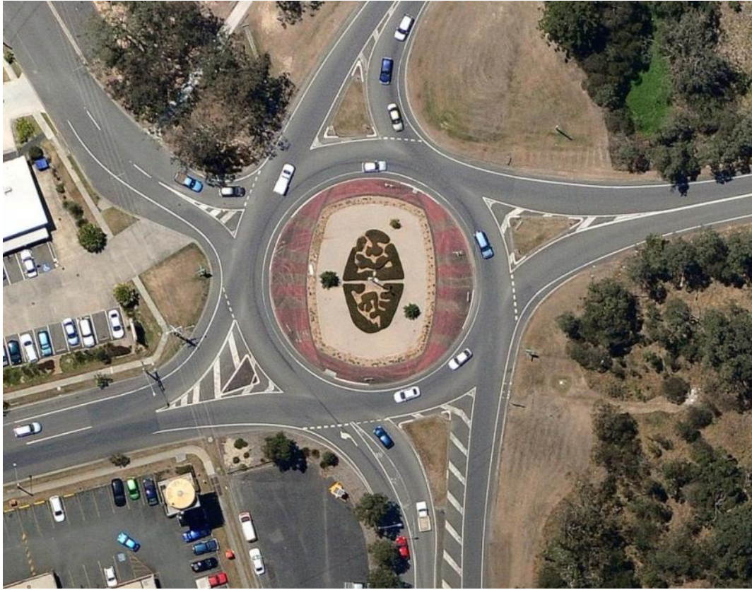
Figure A.1: Example of a Single-lane Roundabout with Five Legs, Burpengary, QLD
