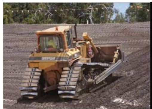
Dozer tracking up batter slope
