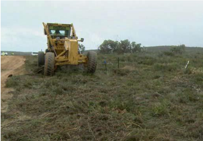
Site topsoil ready for removal and stockpiling
