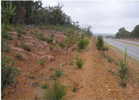
Benching of batter slope.
