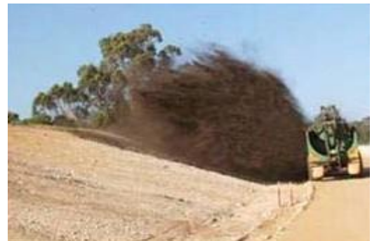
Side spreader of topsoil or mulch
