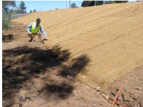
Use of coir matting used to stabilise batter
