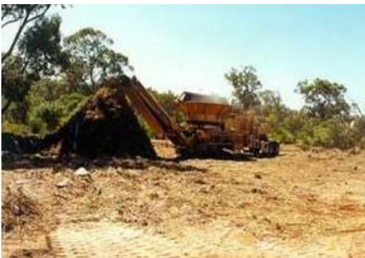
Chipping of site vegetation prior to stockpiling
