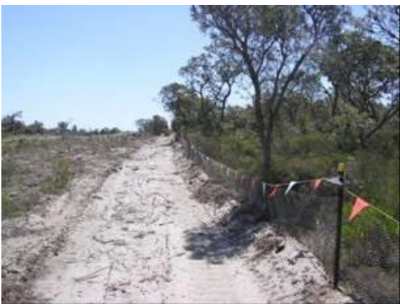
Extent of clearing work clearly pegged on site
