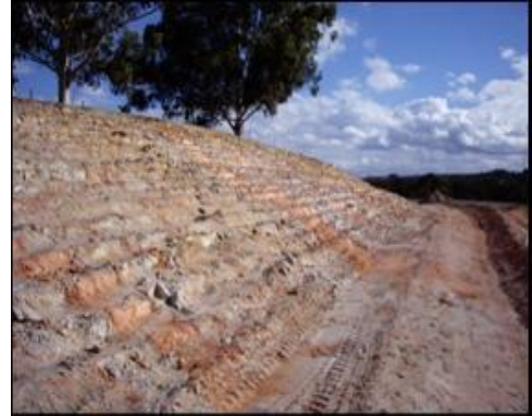
Stepping of batter slope.
