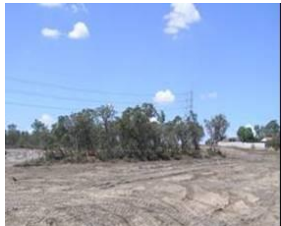
Remnant native vegetation retained and protected within the clearing area.
