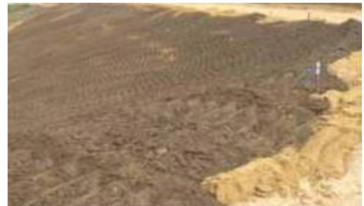
Site topsoil respread over finished batter
