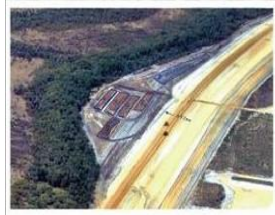
View of constructed topsoil stockpiles within project area
