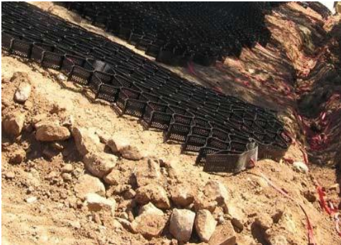
Use of geocell material to stabilise steep batter
