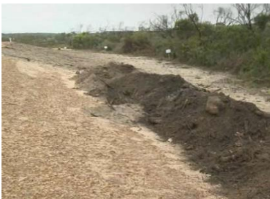
Site topsoil graded into windrow
