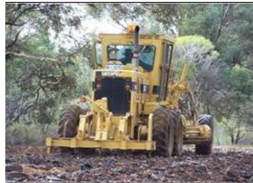
Ripping of redundant pavement area prior to seeding and planting
