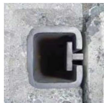
T-Lok coupling system
