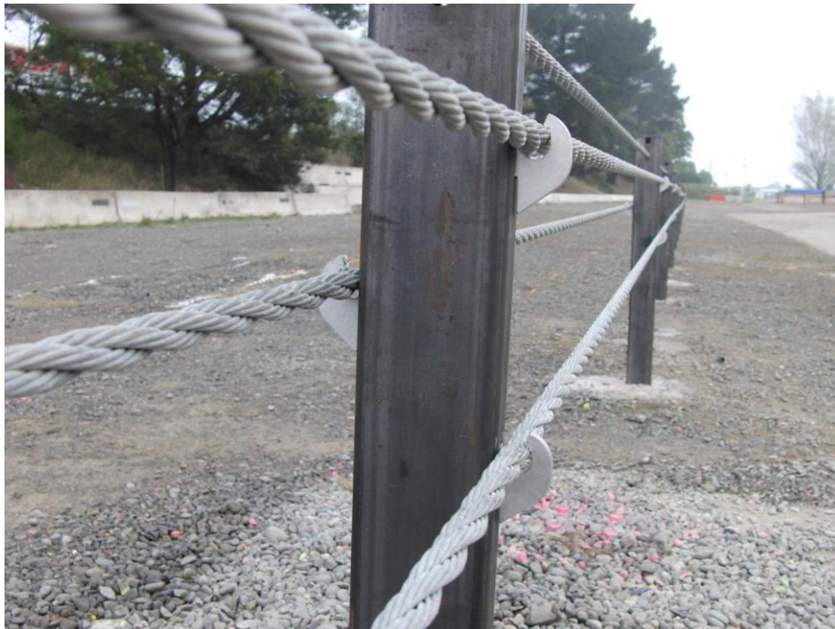
Photograph of Sentryline-M wire rope safety barrier installation.
