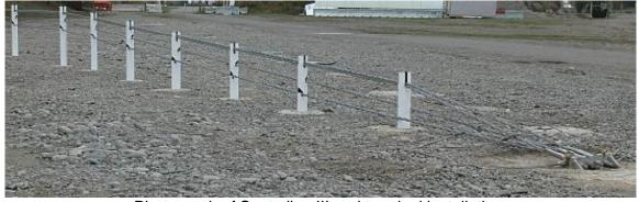
Photograph of Sentryline III end terminal installation.
