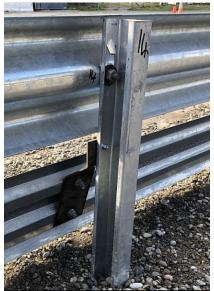
Rear view of RiderPro connected to Sentry W-Beam
