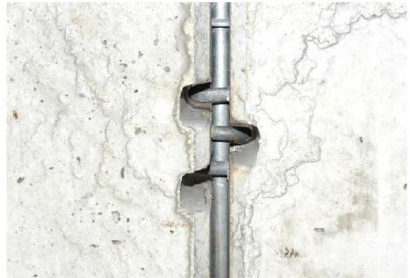
Photographs Pin and Loop Connected Units and Joint
