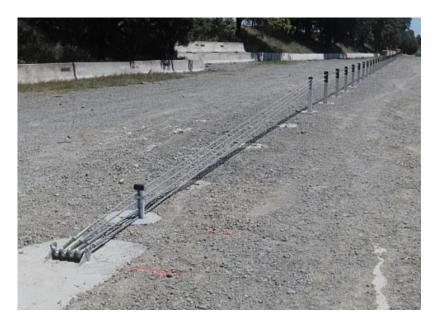
Photograph of installed MashFlex TL3 End Terminal
