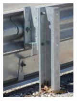
Photo 1: HIASA Rail Rolled End Section
