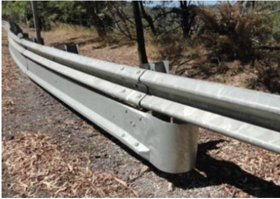
Photo 1: HIASA Rail Rolled End Section
