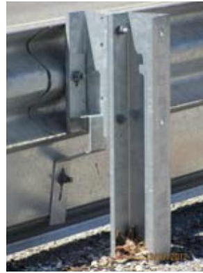
Photo 2: HIASA W-Beam connection
