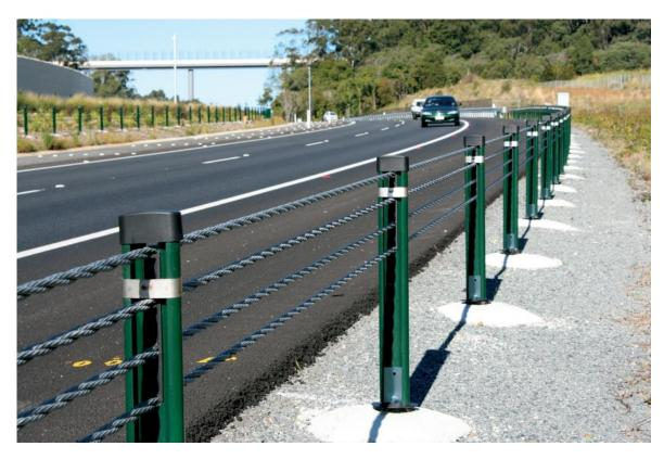
Photograph of installed Flexfence TL4 Wire Rope Safety Barrier
