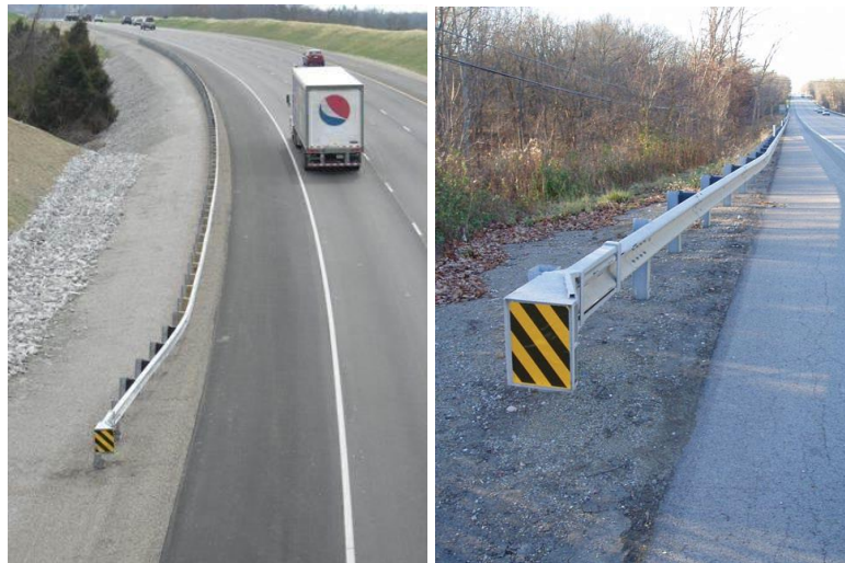
Photographs of FLEAT – SP installations
