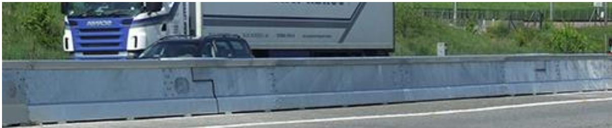
Photograph of BG800 Gate installation
