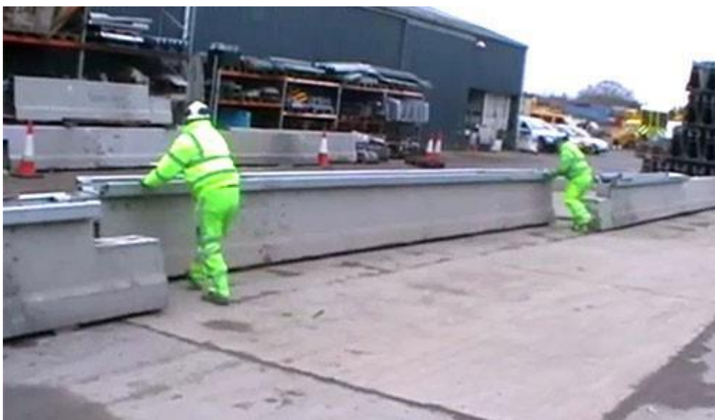
Photograph of BG800 Gate opening
