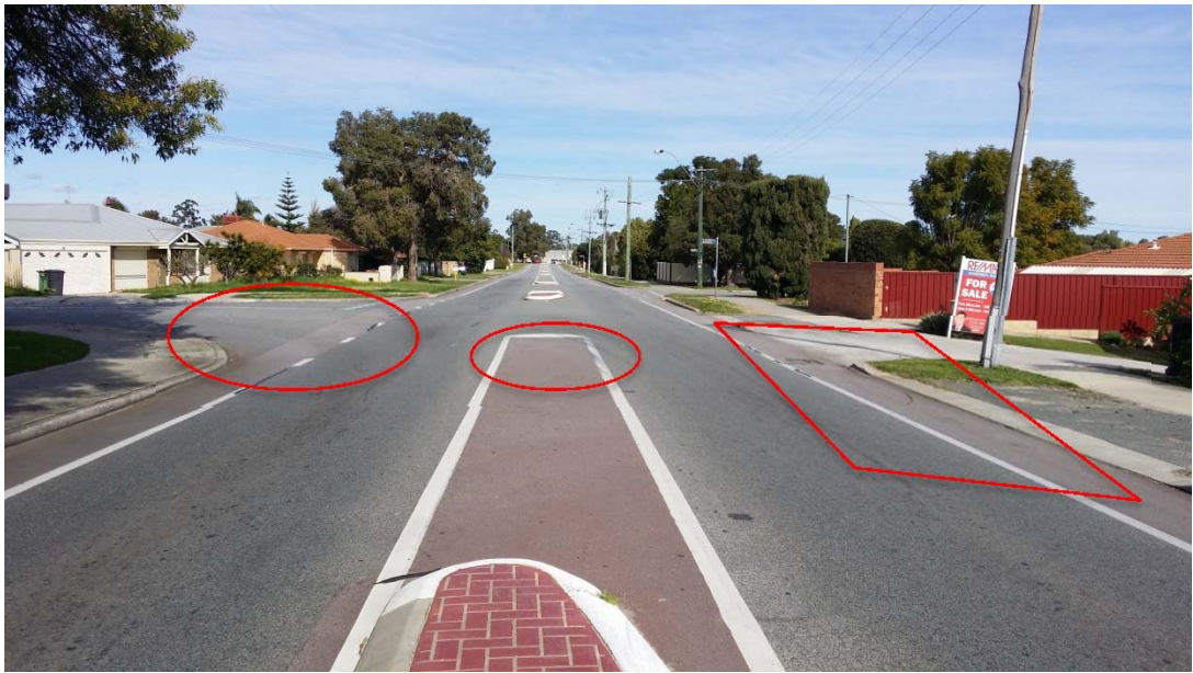
Figure 5 – Median and Shoulders Using Dense Graded Granite Mix with Red Oxide
