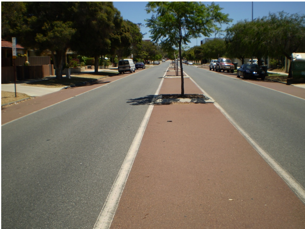
Figure 4 – Median and Parking Bays with Dense Graded Laterite Asphalt
