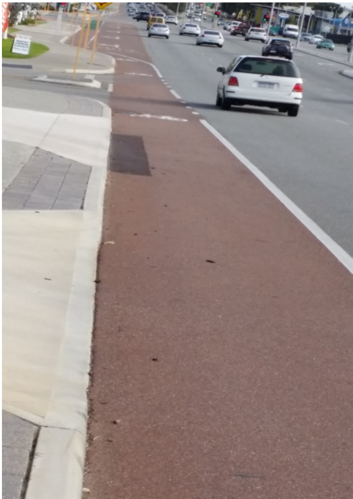
Figure 3 – Cycle Lane with Dense Graded Laterite Asphalt
