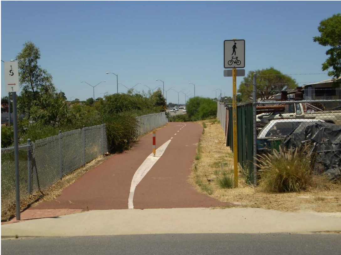
Figure 6 – Shared Path with Dense Graded Laterite Asphalt
