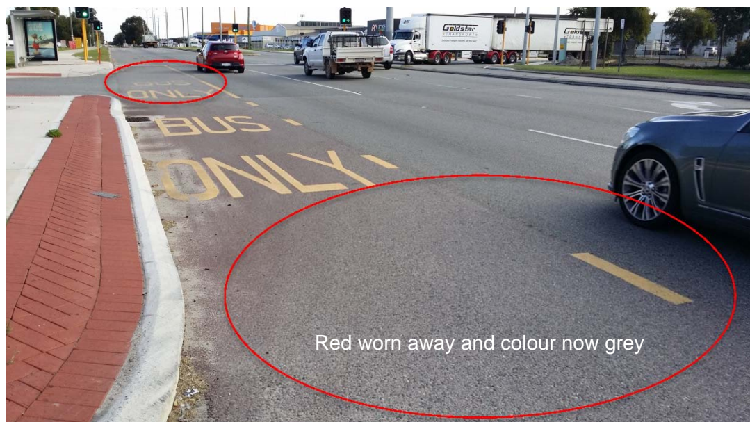
Figure 2 – Dense Graded Granite Mix with Red Oxide
