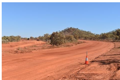
Some sections of Tanami Road will be realigned to improve safety and avoid areas of cultural significance.
