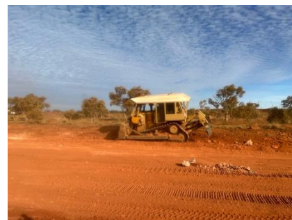
Widening of the road is underway.
