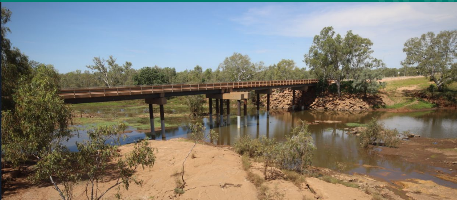
Above: The existing Brooking Channel Bridge.
