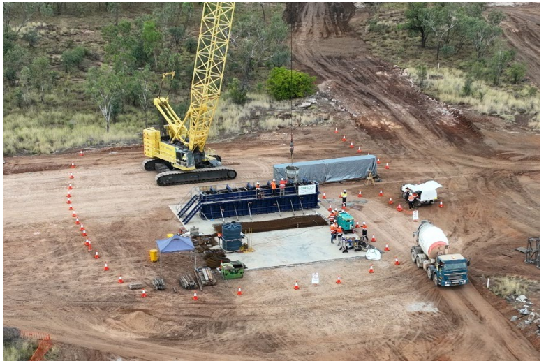
Above: On-site fabrication of the pier shells.
