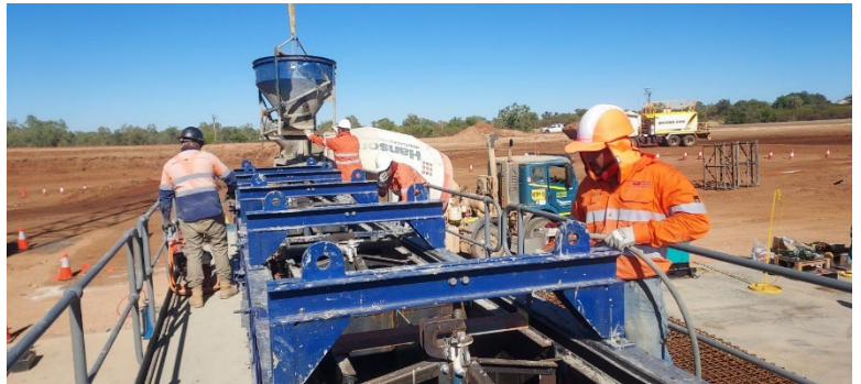
Above: Construction trainee Kevin completing pier shell works.
