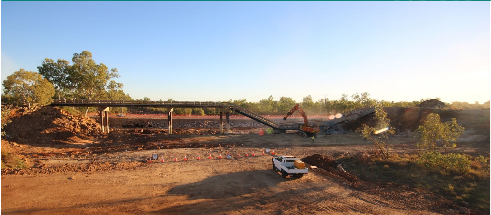
Above: Brooking Channel Bridge demolition works.
