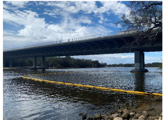
Example of silt curtain
