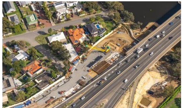
Example of a casting bed next to residential properties
