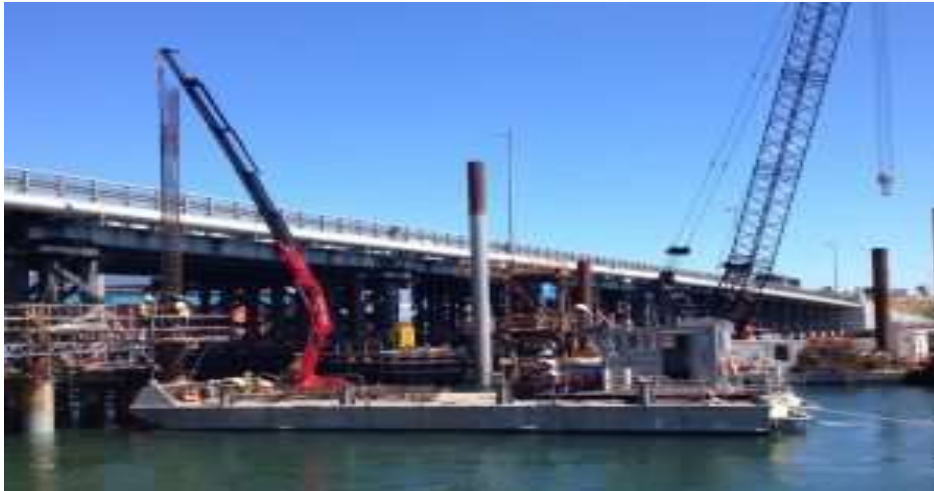
Figure 10 Project marine barge used by IPS
