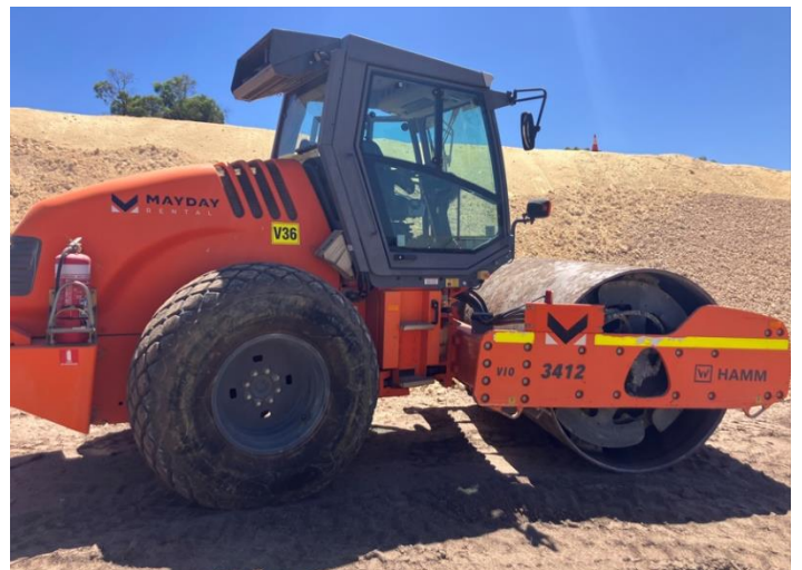
Above: A roller operating on site may cause vibrations when in use.
