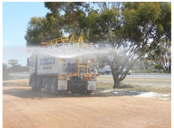
Water application using a water cart.
