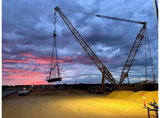
Bottom left and above: Four, 100 tonne beams for the new Walgoolan Bridge are lifted into place. Below: The new bridge takes shape.
