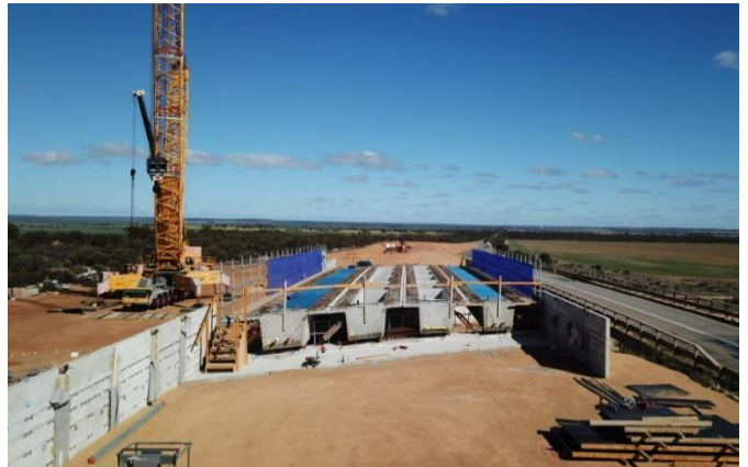
Bottom left and above: Four, 100 tonne beams for the new Walgoolan Bridge are lifted into place. Below: The new bridge takes shape.
