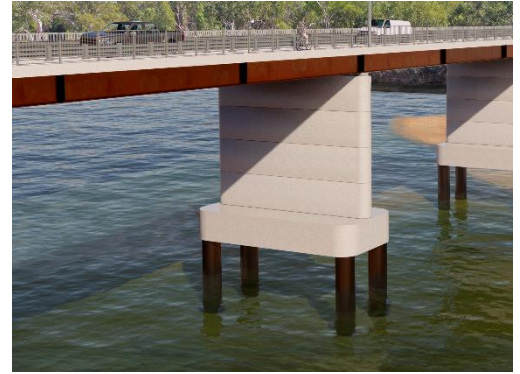
Right: Artist's impression of the pile caps and piers on the New Fitzroy River Bridge.
