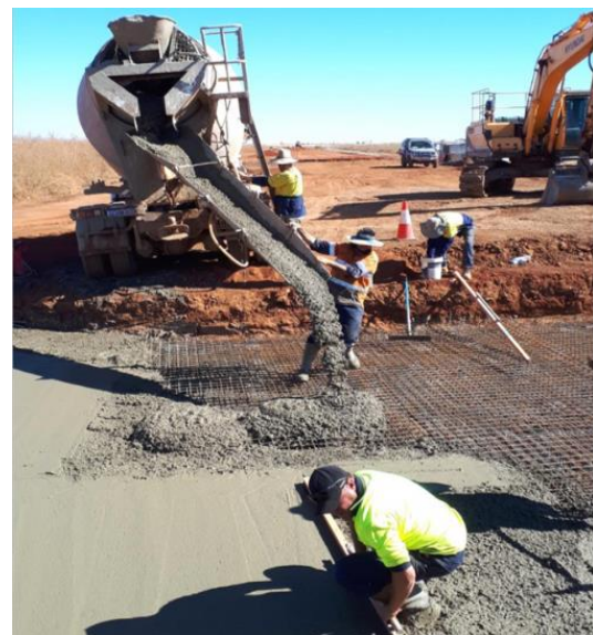
Pouring of culvert base slab, Sturt Creek Crossing upgrade, September 2020
