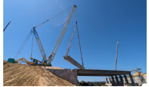
Image Link: RR Beams Mid Lift.jpg
