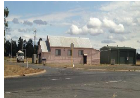
Elgin Hall, with shed for fire-fighting equipment attached
