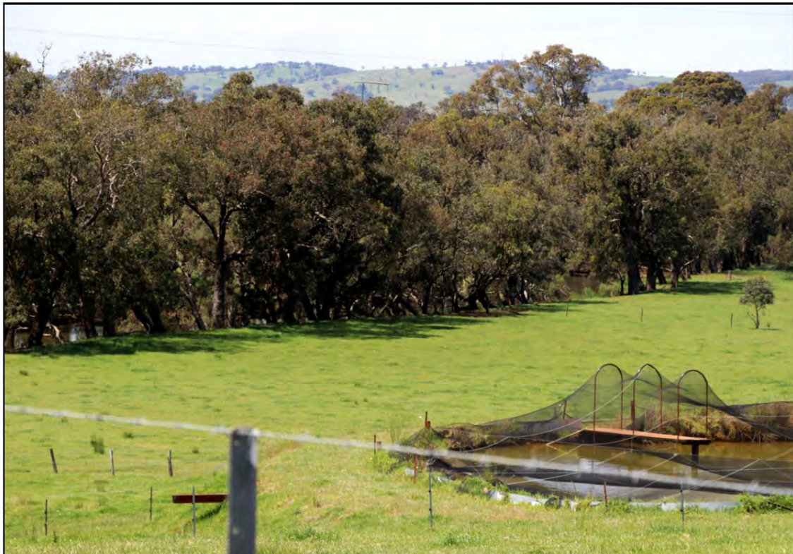
Figure 7: The location of the proposed Bridge 1839 & 1840 over the Collie River accessed via Clifton Road between Lot 121 and Lot 424 at coordinates 385475mE 6314596mN; view looking north-east.
