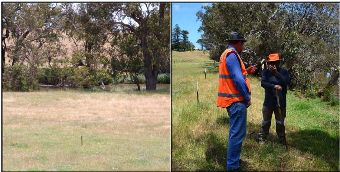
Figure 13: left pegs showing the corridor line and abutment location. Right Mr McCarthy and Mr Northover discuss the project with the pegs behind.
