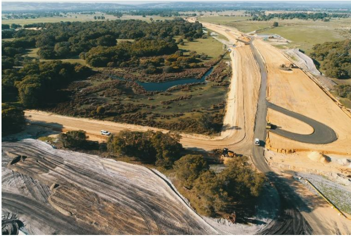
Work underway at the Forrest Highway project site
