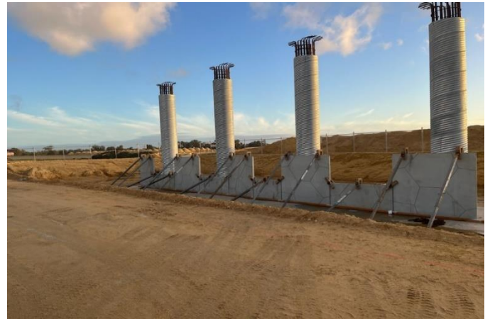
Installation of the mechanically stabilised earth (MSE) walls at Raymond Road
