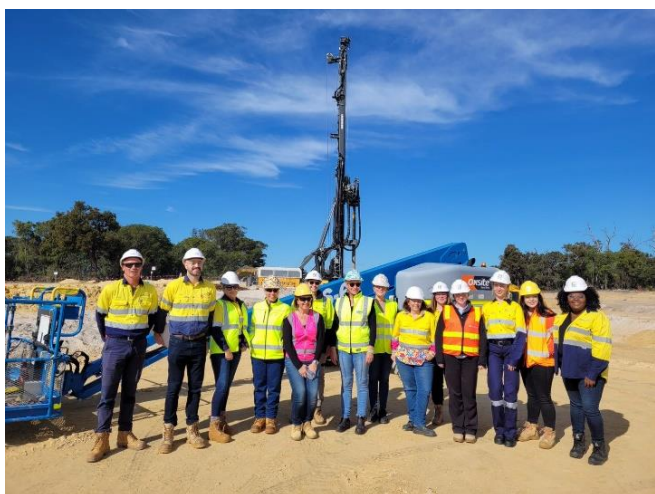
NAWIC members on-site at Forrest Highway
