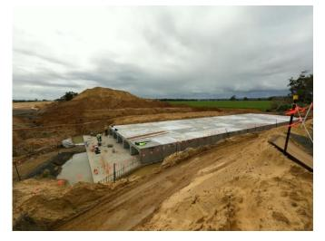
Concrete box culverts being installed on top of the concrete slab at the Raymond Road construction site
