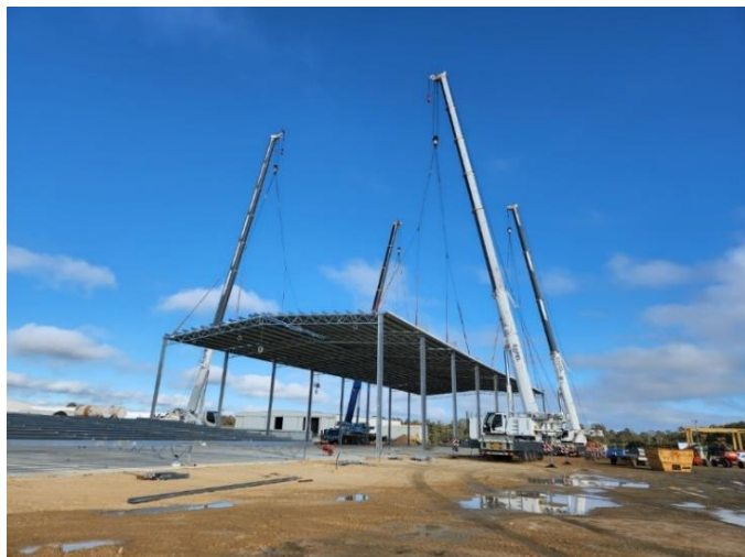
Main shed in the pre-cast yard being erected
