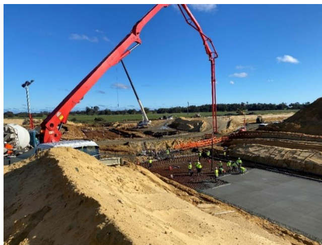
Concrete pour works occurring near Raymond Road
