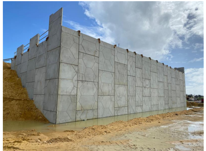
Installation of pre-cast panels at Raymond Road with tortoiseshell design
