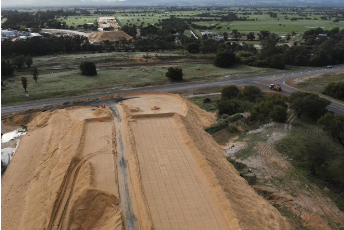
The 'mega-bridge' under construction near Golding Crescent
