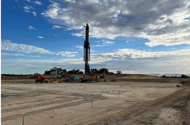
Drill rig at Raymond Road site
