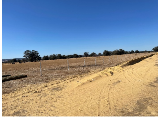
Fencing installation at the South West Highway project site
