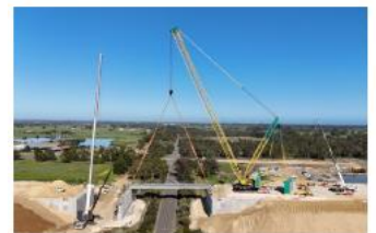
Railway Road Bridge
