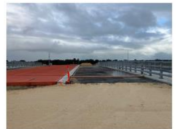
Raymond Road Interchange
