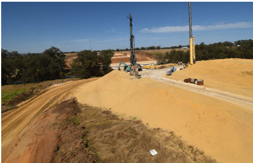
The piling rig working at one of the Collie River bridges
