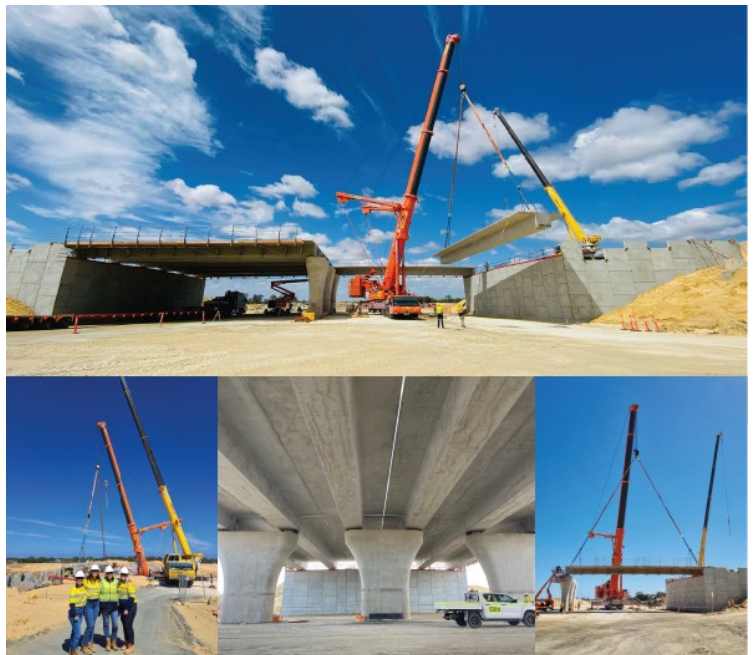
Bridge beams being installed at Raymond Road construction site
