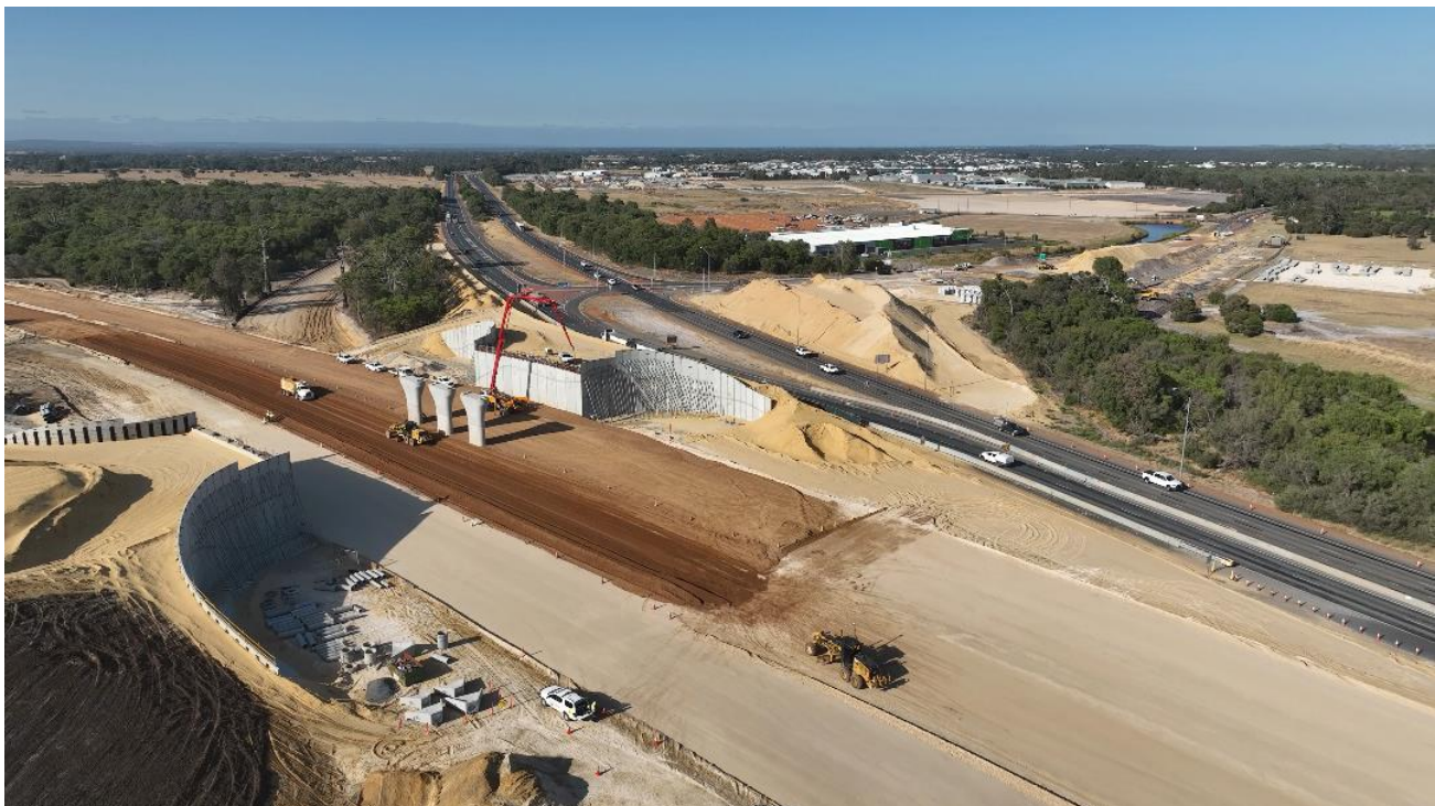
Activities onsite at the Paris Road and Clifton Road interchange
