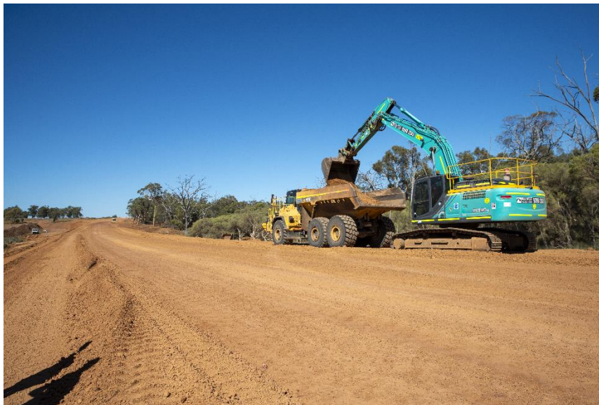
Early works underway, creating local employment opportunities
