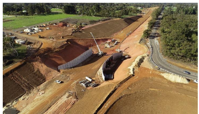
South Coast Highway bridge site
