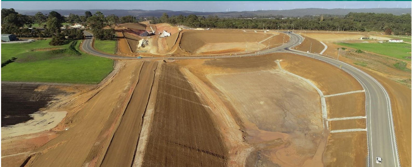
Temporary realignment of South Coast Highway and construction of the interchange
