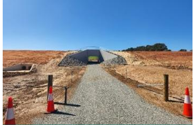
Shared Path and underpass open to the community
