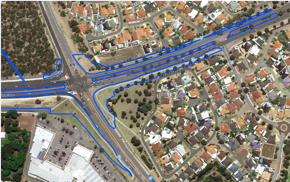
Joondalup Drive and Wanneroo Road intersection
