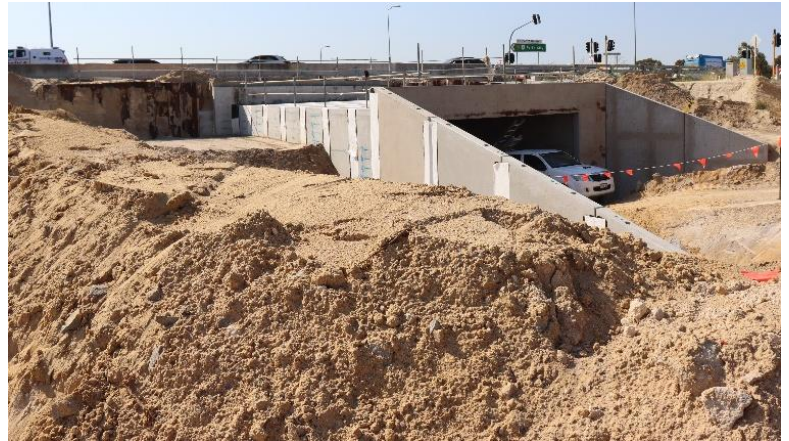
Great Eastern Highway underpass
