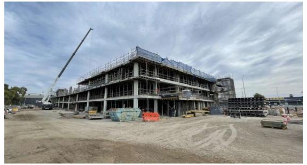
Morley Station multi-storey car park progress
