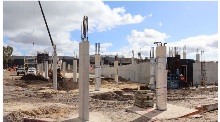
Morley station multi-storey carpark
