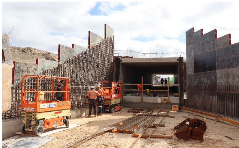
Benara Road underpass
