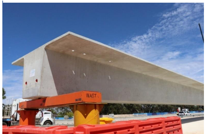
Broun Avenue bridge beams
