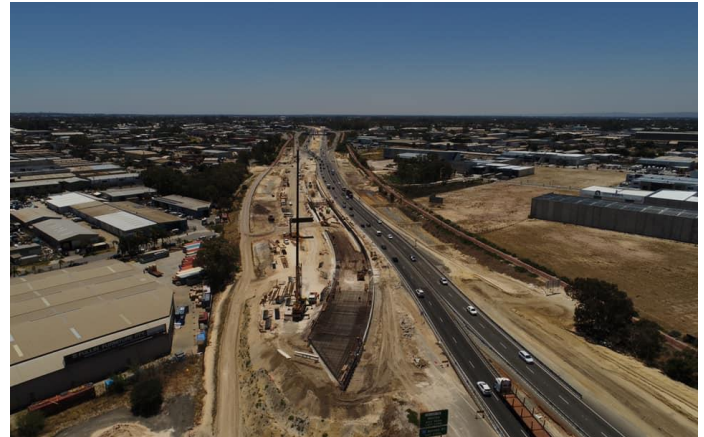
Progress at the Southern Dive
