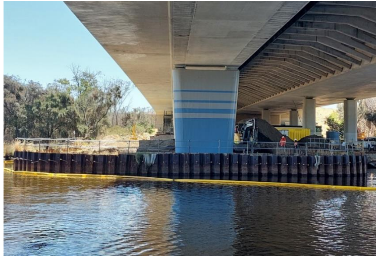
Cofferdam removal at Redcliffe Bridge
