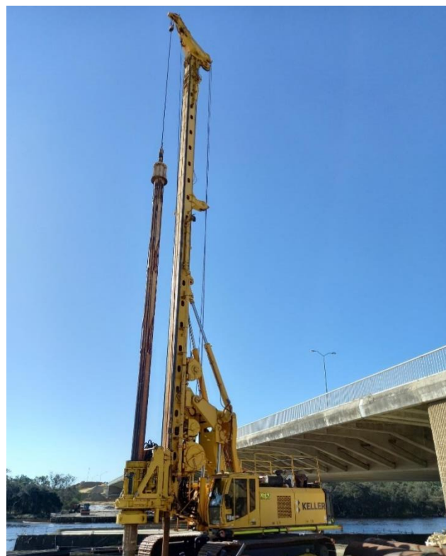
Piling rig at the southern foreshore of the Redcliffe Bridge site.
