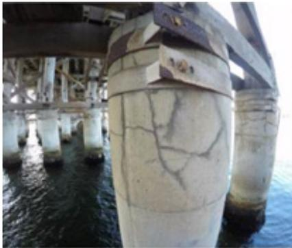
Cracks in concrete encapsulation due to reinforcement corrosion
