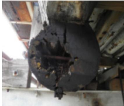
Multiple corbels split and large areas of deterioration/section loss
