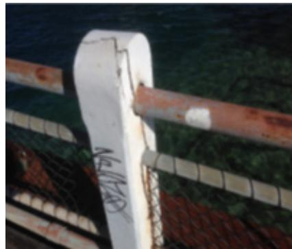
Pedestrian path too narrow, balustrade too low and in poor condition – high risks for cyclists using the shared path
