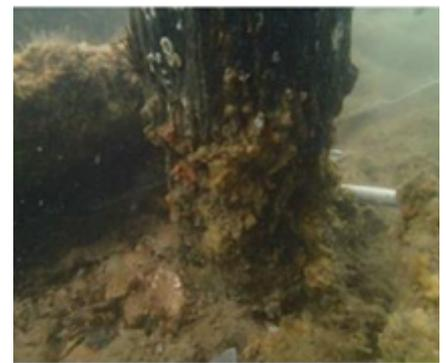
Exposed timber piles at river bed level – noticeable “necking”
