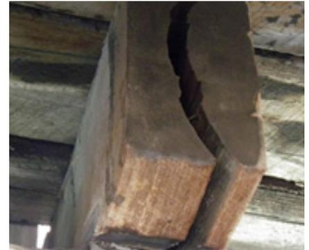
Poor condition of timber deck and timber bearers
