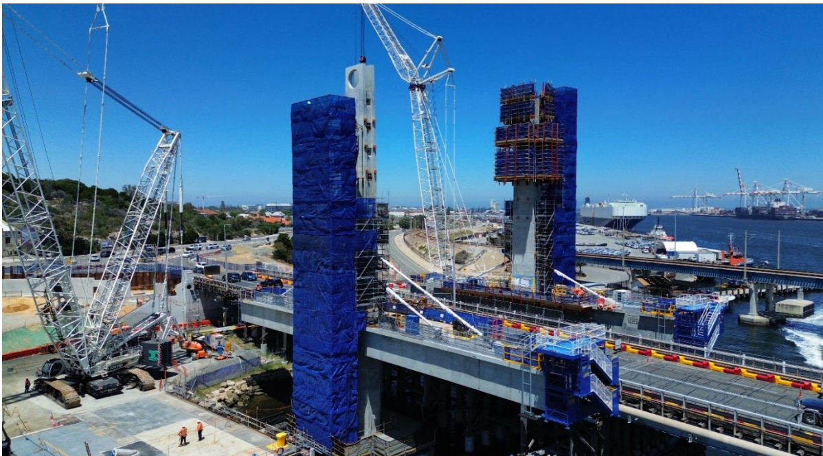
Figure 5: Completed southeast tower.
